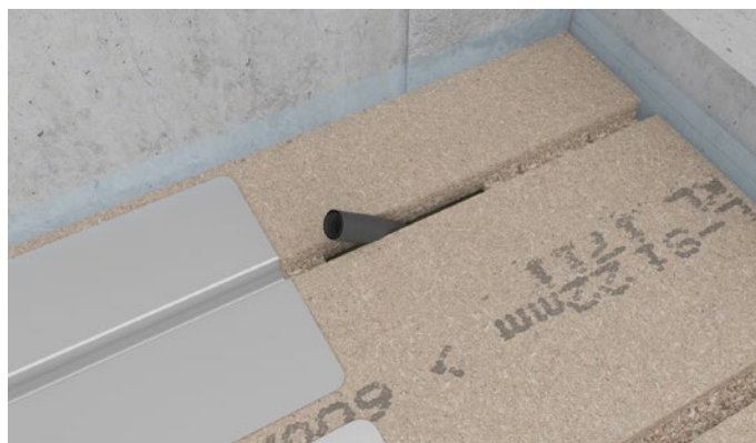
Figure 7 Check that the end of the tube is level with the floor panel.
