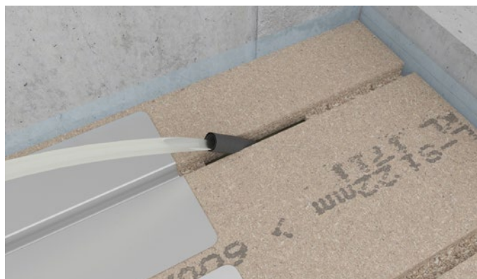
Figure 9 Insert the heating pipe through the empty tube and place it in the grooves on the Climate Floor.
