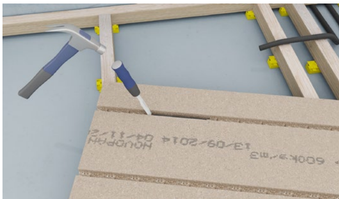
Figure 4 Cut the hole clean with a chisel.
