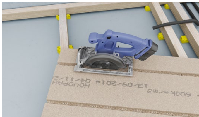
Figure 3 A hole of 15-20 cm is cut in the bottom of the groove on the Climate Floor at the point where the tube will come up through the floor.
