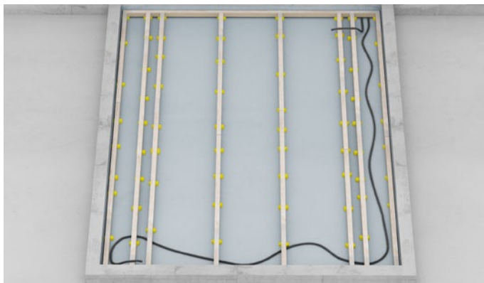
Figure 2 The conduit tube is installed under the floor joists and secured before installing the Climate Floor panels.
