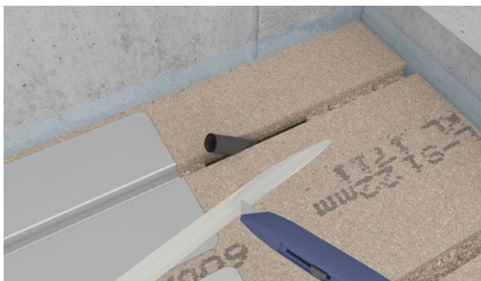
Figure 8 The heating pipe can be sharpened with a knife to facilitate insertion into the tube.
