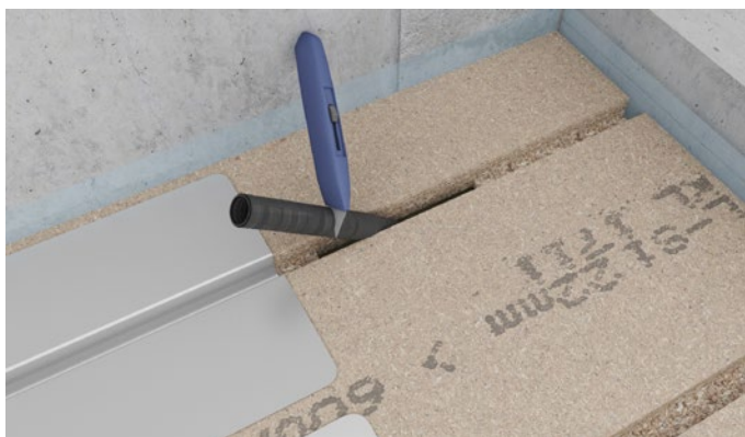
Figure 6 Cut off the excess part of the conduit tube.
