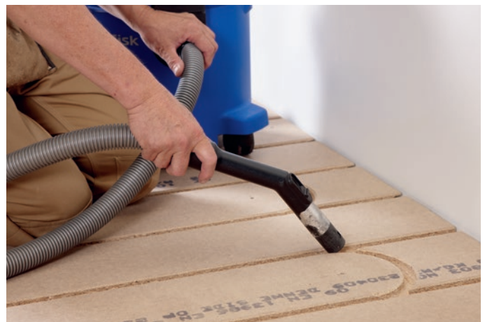
Figure 8 Careful cleaning prevents squeaking noises.
