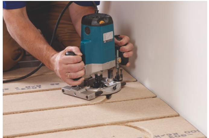
Figure 7 Cutting turning grooves in every 2nd row.
